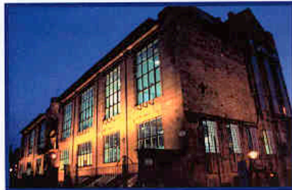
Glasgow School of Art, 1897-1907 Designed by Charles Rennie Mackintosh [Building Services Heritage, B M Roberts, 2003]
