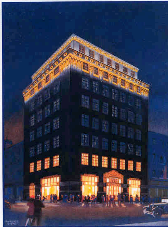
The National Radiator Building (Ideal House), London, 1928 Designed by Raymond M Hood & Gordon Jeeves [Art Deco Architecture, Patricia Bayer, 1992]
