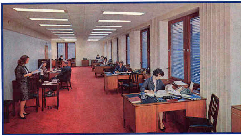
Shell Centre, London, 1962 [International Lighting Review, XIII, 6, 1962]
