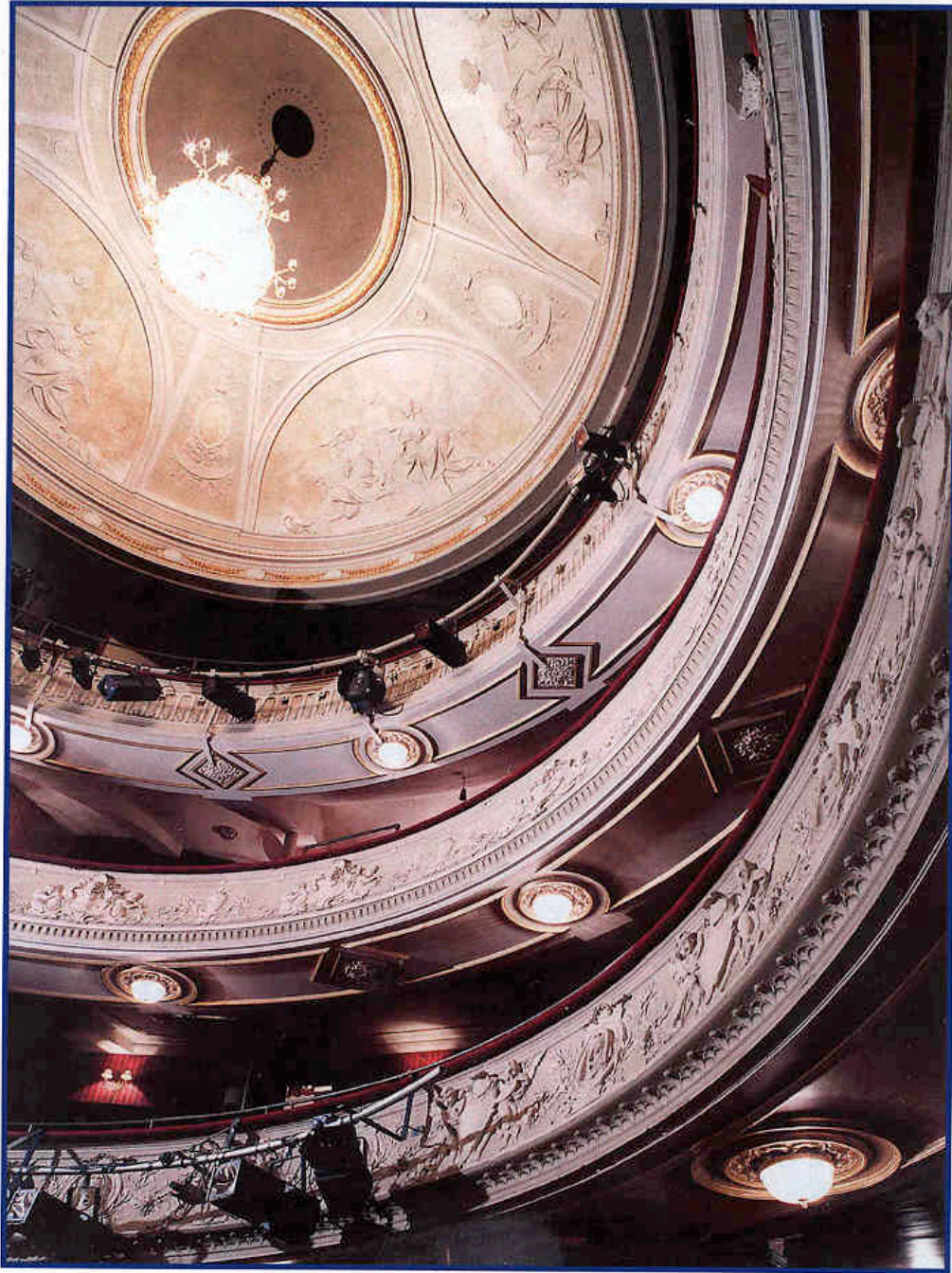
The Garrick Theatre, London, Charing Cross Road, London, 1889 Now with lighting bars across the balcony fronts Architect Walter Emden with C J Phipps. [Scene/Unseen, English Heritage, 2003] [Photograph National Monuments Record, AA020204]
