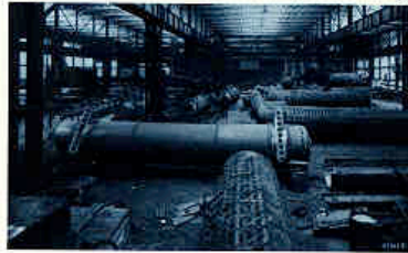
Water Tube Boilers in the 1920's
