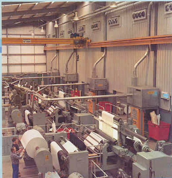
A waste recovery installation.
