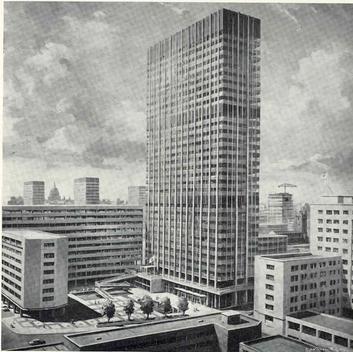
BRITISH PETROLEUM HEAD OFFICE BUILDING, LONDON This building, forming part of the London Barbican scheme, consists of two low-level blocks and a 30-storey tower block. 3500 induction units are used to air condition the perimeter rooms of the tower block; other areas use high velocity dual-duct, and traditional low velocity systems. Four water tube boilers give a total heat output of 52 MBtu/h, and the cooling power of the refrigerating plant totals 1750 tons. Architects: Joseph F. Milton, Cashmore & Partners. Consultants: G. H. Buckle & Partners. Main contractor: John Laing Construction Ltd.
