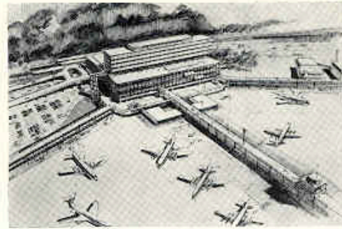
LONDON (GATWICK) AIRPORT EXTENSION.
