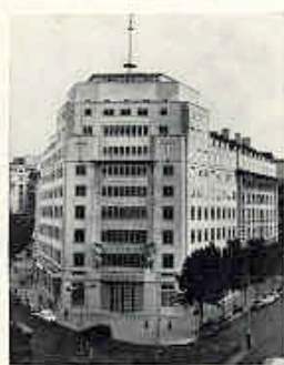
ENGLISH ELECTRIC HOUSE GAIETY SITE, LONDON This building is air conditioned throughout by a dual-duct high velocity air system.
