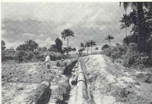
MICHELIN (NIGERIA) LTD., PORT HARCOURT, NIGERIA. Services provided by Brightside include air conditioning, ventilation, compressed air, process refrigeration plant, and all piping services throughout the factory. The refrigeration plant consists of two centrifugal machines with a total capacity of 880 tons of refrigeration. Condenser cooling water was piped through 2½ miles of jungle in 24 in and 16 in diameter tubing. Consultants: Michelin Tyre Co. Ltd., Stoke-on-Trent.
