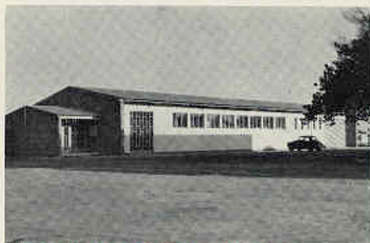
EDUCATION CENTRE, KHORMAKSAR CAMP, ADEN. Air conditioning is provided by a system of high level fan-coil units served with chilled water and ventilation air from a central plant. A packaged chilled water set works in conjunction with a cooling tower. Each classroom is provided with individual thermostatic control. Consultants: Brandt & O'Dell.
