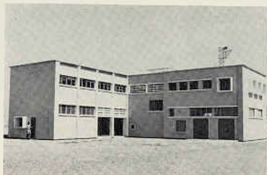
CABLE & WIRELESS LTD. RECEIVER STATION, SALT PANS, ADEN. Packaged air cooled refrigeration air handling units supply conditioned air to communication bays, and administrative offices. The associated transmitting station in this area was also conditioned by Brightside using a similar type of system. Architects: Cable & Wireless Architects Dept.
