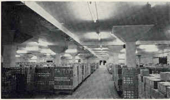
CONFECTIONERY STORAGE & DISTRIBUTION DEPOT, CADBURY BROS. LTD., ILKESTON.
