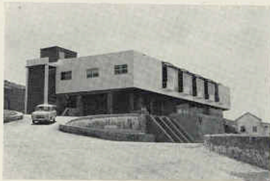
MATERNITY HOSPITAL, STEAMER POINT, ADEN. Operating theatres and delivery rooms are conditioned by a 100% fresh air plant with humidity control. Ward areas and corridors are conditioned by self-contained units conditioners with overhead distribution. Consultants: Brandt & O'Dell.
