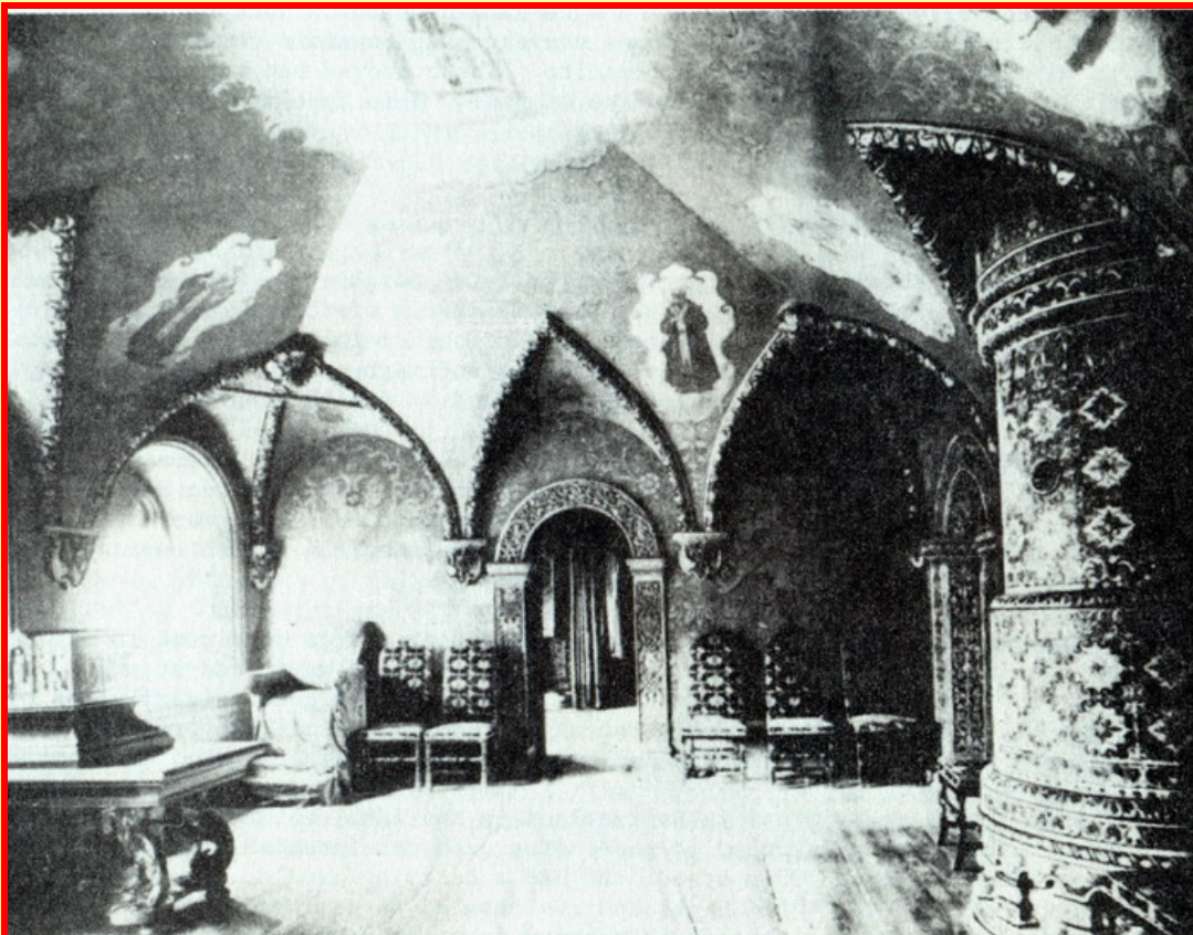
Fig. 3.7 A room in a Moscow palace, showing a large heating stove built into one wall and serving two adjacent rooms. (Courtesy Shell-Mex)
