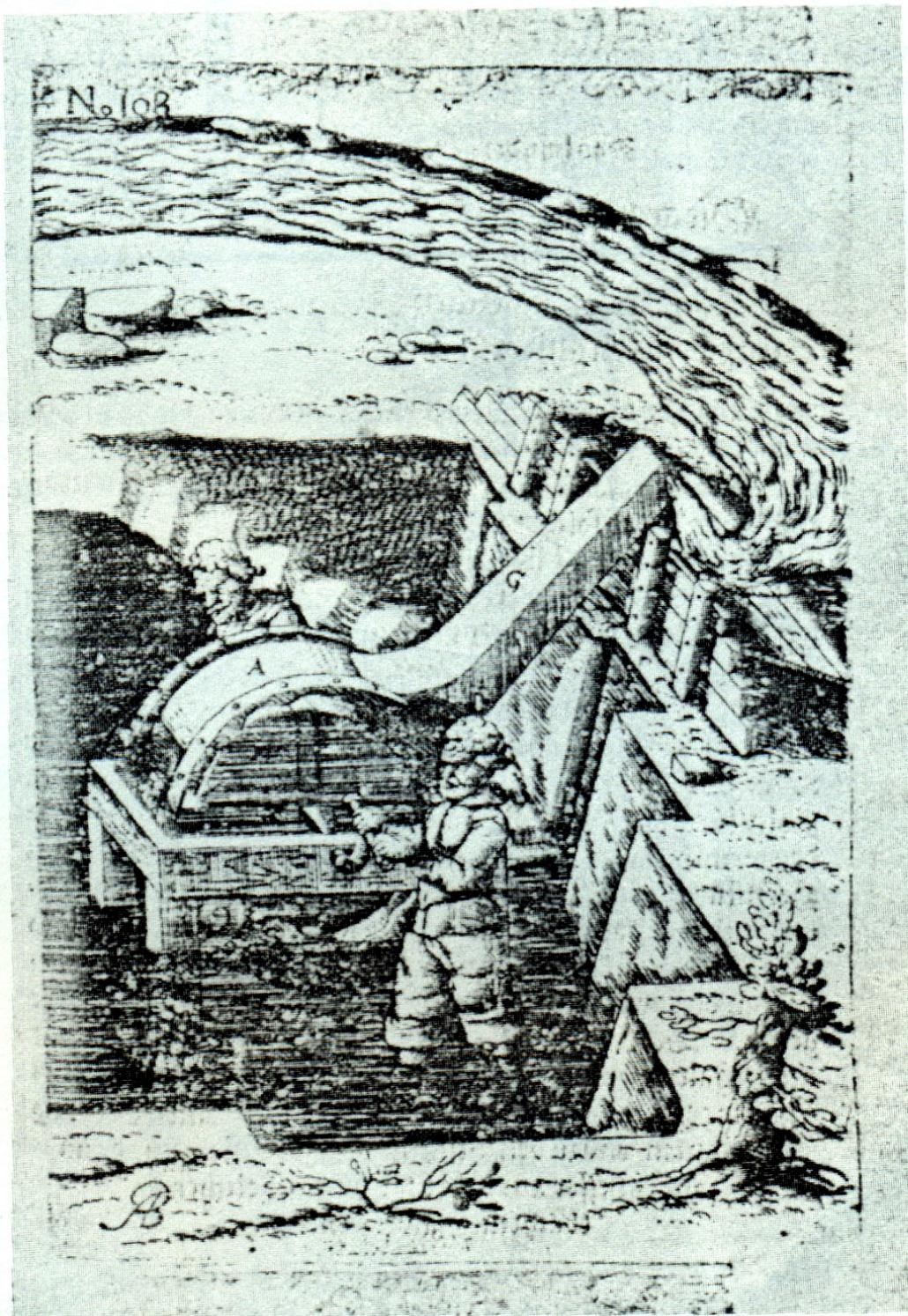
Fig. 8.5. Rotary displacement pump (from Ramelli, 1588).
