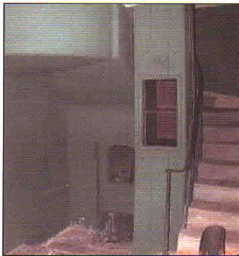
Haden stove of 1826 in situ
