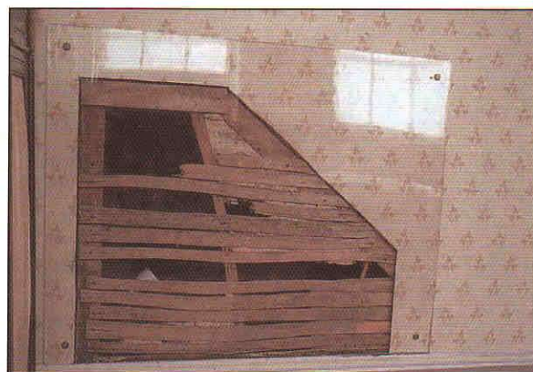
Cut-away wall section with hot air duct behind
