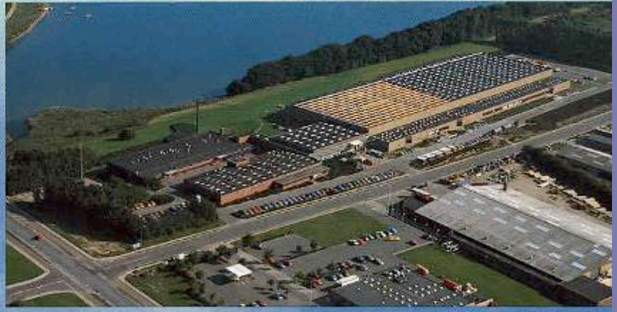
Electrical and electronic products are made here at the factory in Graasten.
