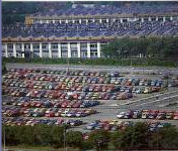
A section of the factory viewed from across one of our car parks.
