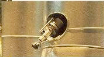
▲ For invoicing, metering and monitoring in a power/heating station there are Danfoss ultrasonic flow transmitters.
