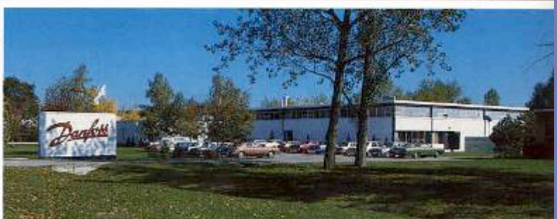
Danfoss Manufacturing Company Ltd., Mississauga, Toronto, Canada.
