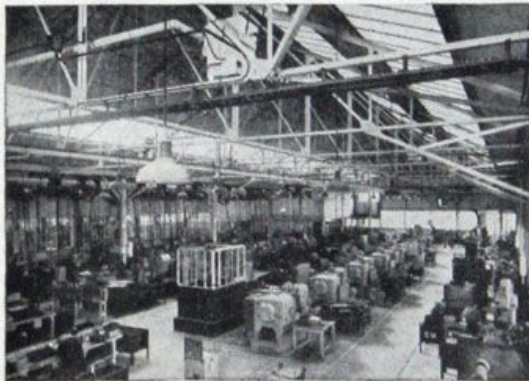
General view of the Crane Gun Metal Valve Machine Shop.
