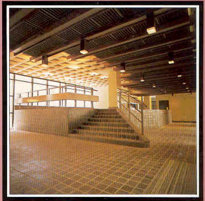
Above / Registrar General Building, Mauritius / Photos show a section of staircase and bar in the Banqueting Hall and part of the main plant room within the complex where Drake & Scull was awarded the design and installation of all mechanical, electrical, public, fire protection and air conditioning services.
