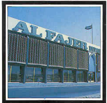
Above / Al Fajer Department Store, Dubai, U.A.E. / The electrical contract completed by Lunar Drake & Scull (U.A.E.) comprised the installation of general lighting, standby generator systems and fire protection systems for this 19 department, two-storey department store, one of the biggest of its kind in the U.A.E.
