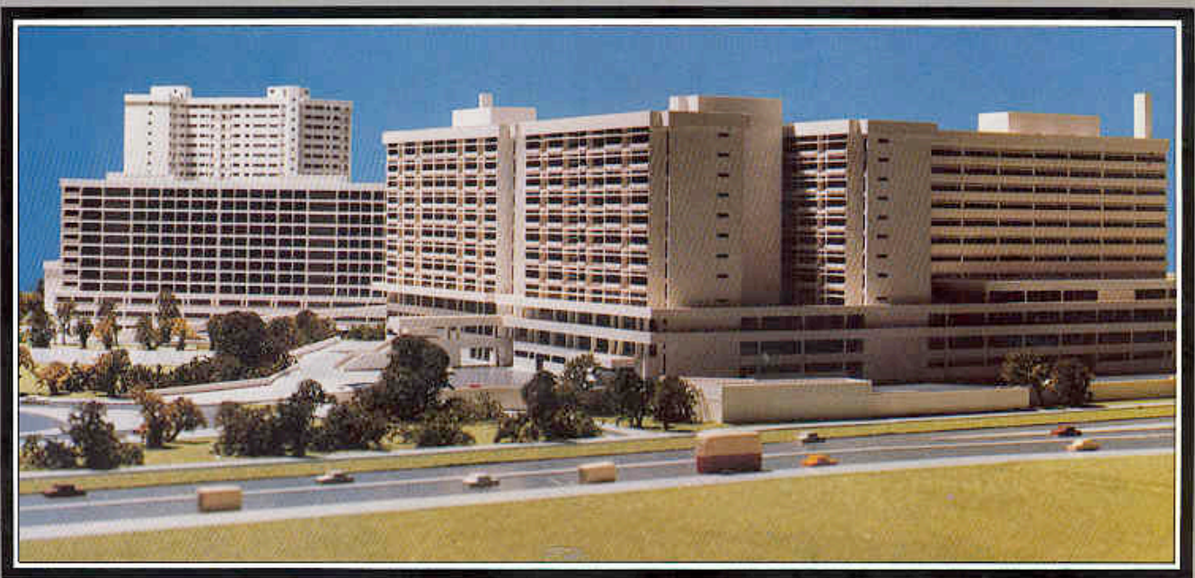
Top / Sun Hung Kai Centre, Hong Kong / Drake & Scull (Hong Kong) Ltd. is responsible for the design of all engineering services for this 50 storey tower complex. Bottom / Sha Tin Teaching Hospital, Hong Kong / Drake & Scull (Hong Kong) Ltd. has been awarded the contract for the installation of all air conditioning, ventilation and steam plant comprising a central chilled water system, central air handling plant and air terminals. When fully completed in 1982 the hospital will have 1400 beds and serve 700,000 people in the eastern area of the New Territories.
