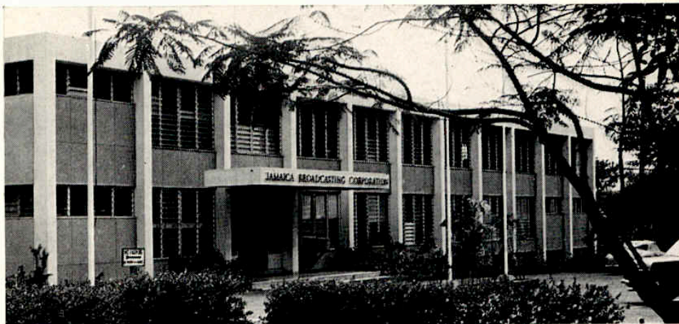
The Jamaica Broadcasting Corporation building in the West Indies, also equipped with Ottermill products.
