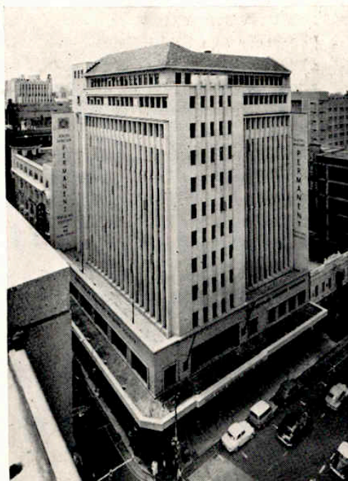
Ottermill rising main equipment is installed in the new building of the South African Permanent Building Society in Johannesburg.
