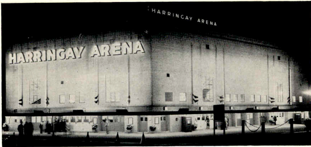
At Harringay Arena the installation was carried out by Drake & Gorham Ltd. Main switchgear was constructed at the Acton factory.
