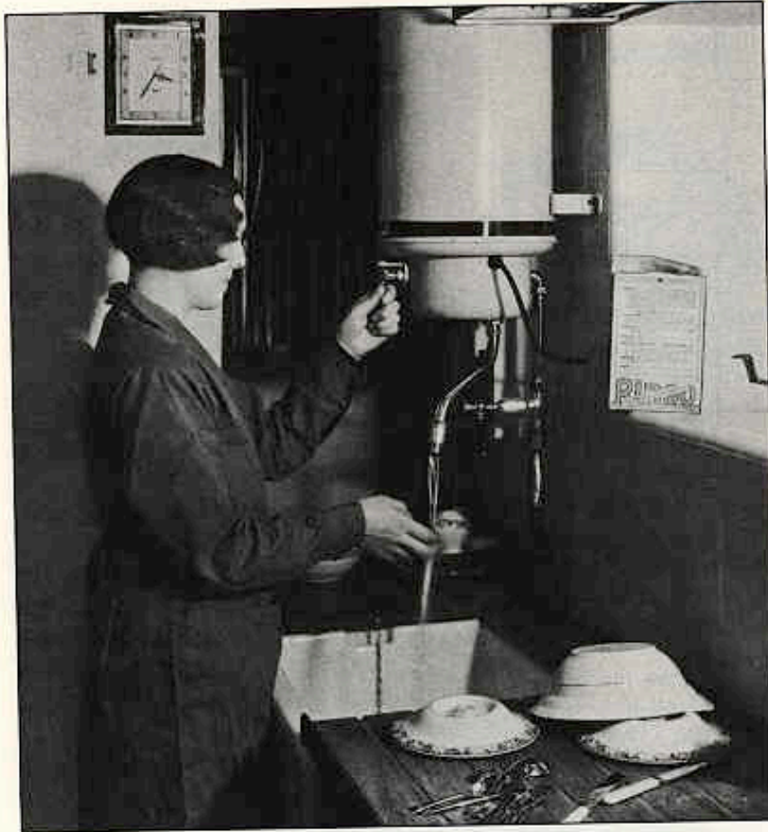
Electric water heating at the sink (1930).
