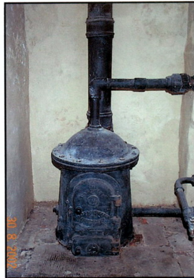
Jones & Attwood hot water Pot boiler, c.1890 discovered at Tyntesfield
