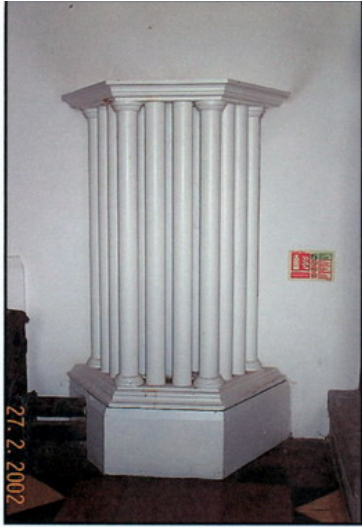
Vertical tubular radiator by Vincent Skinner, Bristol Church of St Andrew, Cheddar
