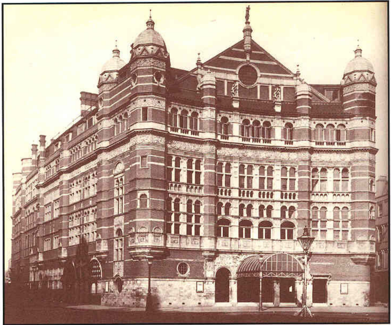
The Royal English Opera House, London, the dream of Richard D'Oyly Carte, built by T E Holloway with architect T E Colcut, 1899. "Far below the stage its own current was manufactured....the electro-motors also supplied the house with fresh air, passed over ice in summer, and hot-water pipes in winter. Stale air was electrically extracted, a very early use of air conditioning." However, it failed commercially and in 1892 reopened as the Palace Theatre of Varieties.
