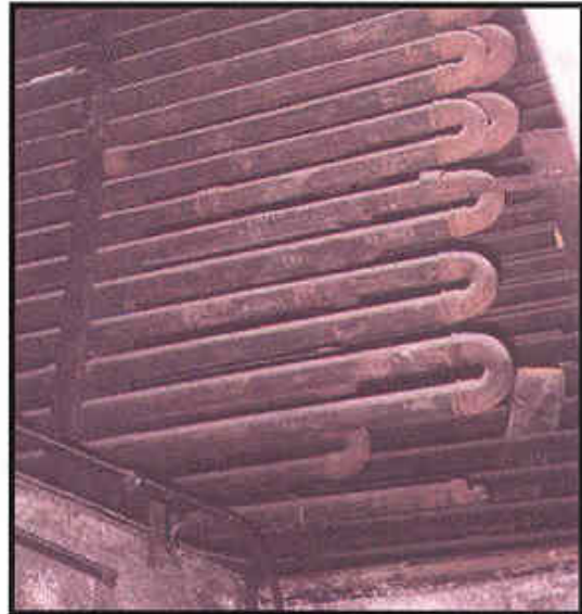
Plain tube hot water air heater coil 1903
