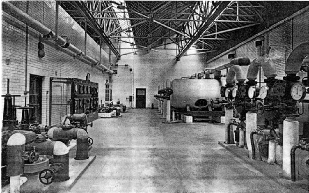
Calorifier and Pump Chamber by Hadens. 50 million B.Th.U. per hour.
