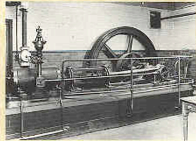
A Haden horizontal steam engine
