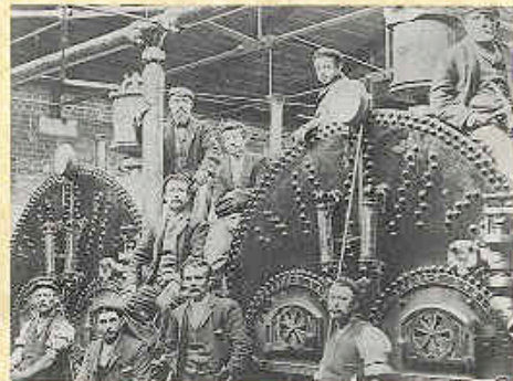
The steam boiler erection team
