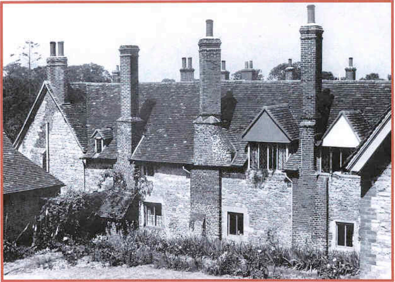
The hospital almshouses. Note the tall chimney stacks, a notable feature of many almshouses, each serving a dwelling, [TCEH, 71]
