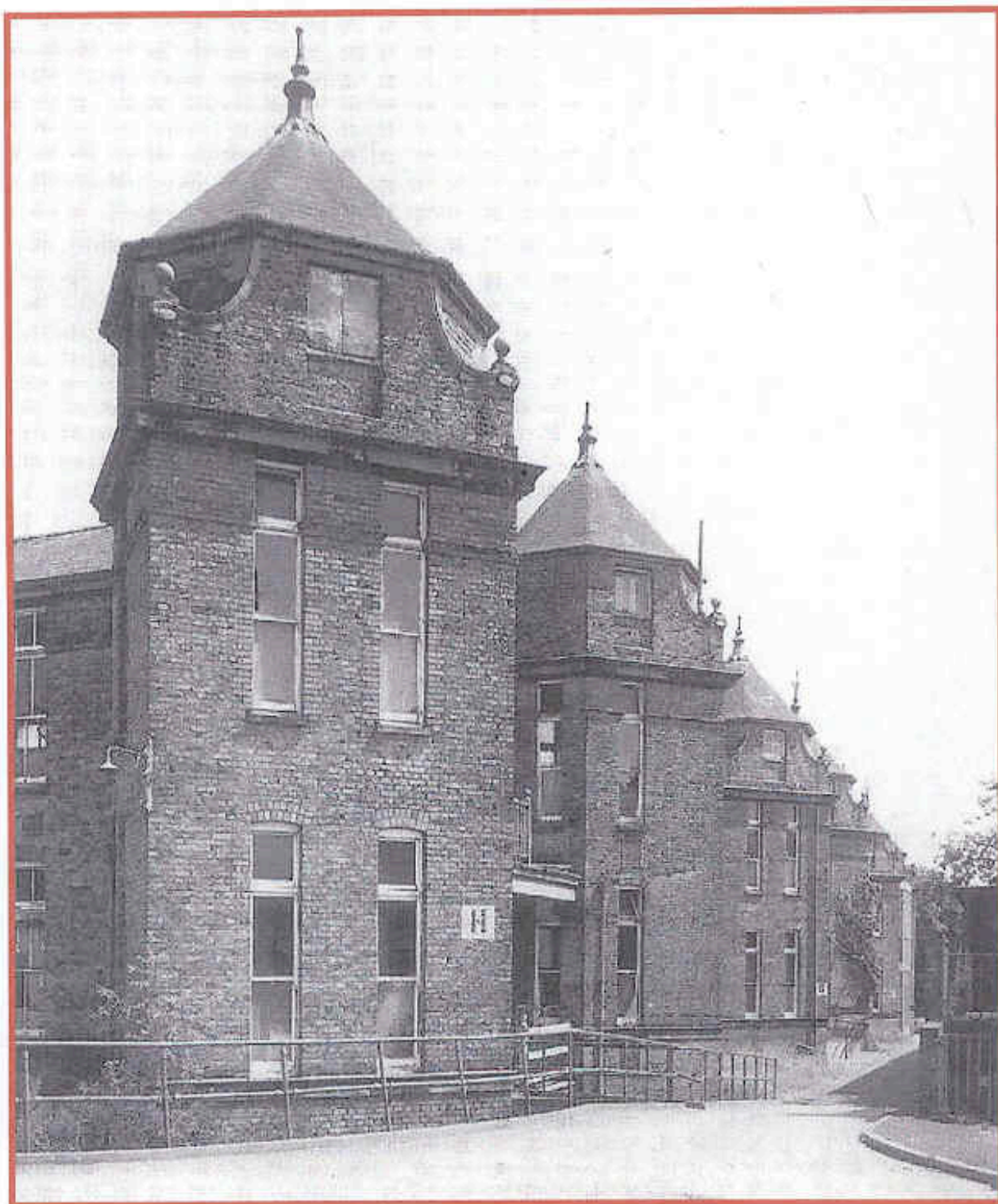
View of sanitary towers at the ends of the ward pavilions, 1897 [EH, 139]
