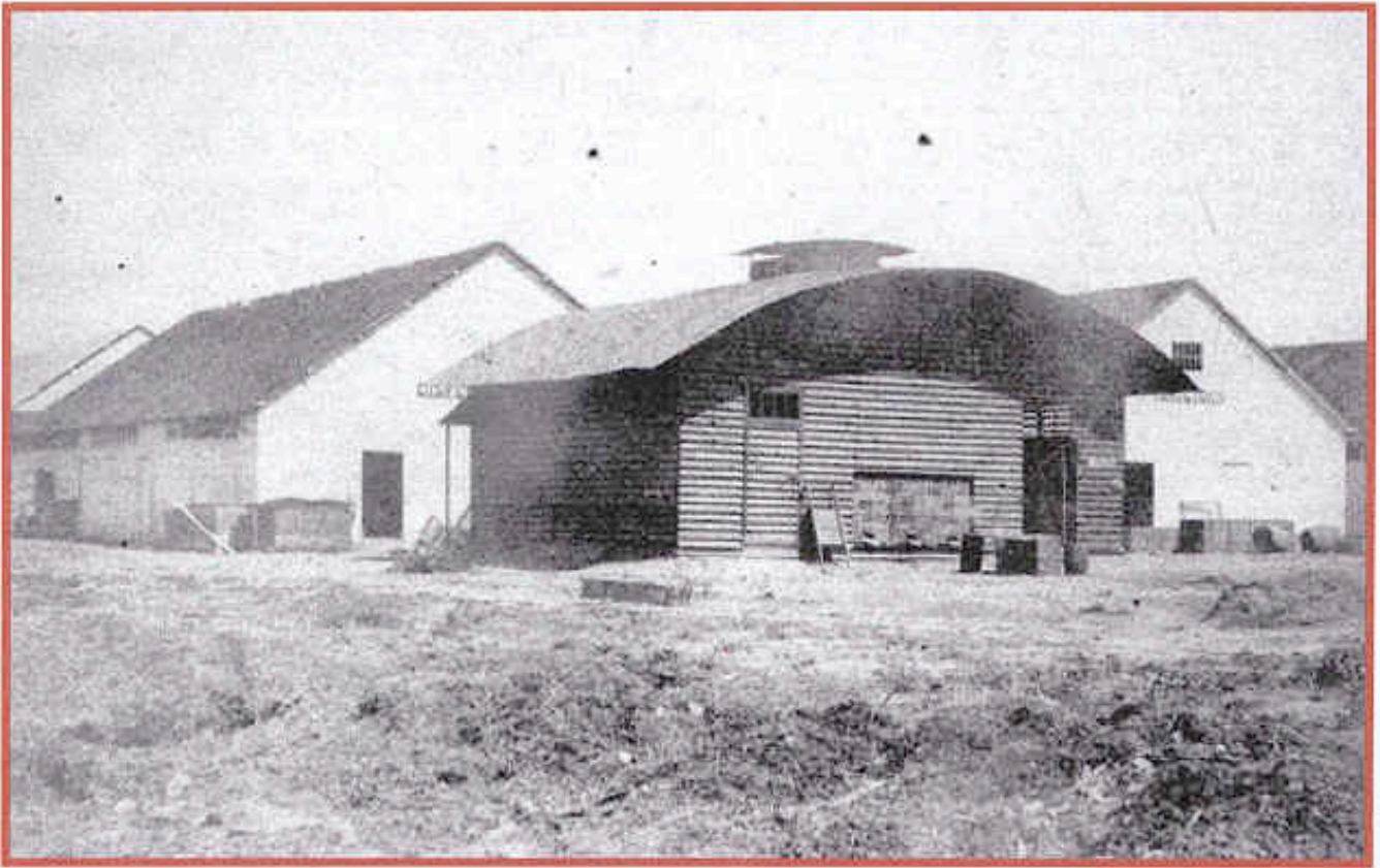
One of Brunel's prefabricated hospital buildings erected at Renkioi in Turkey in 1855-56 [Design Museum]
