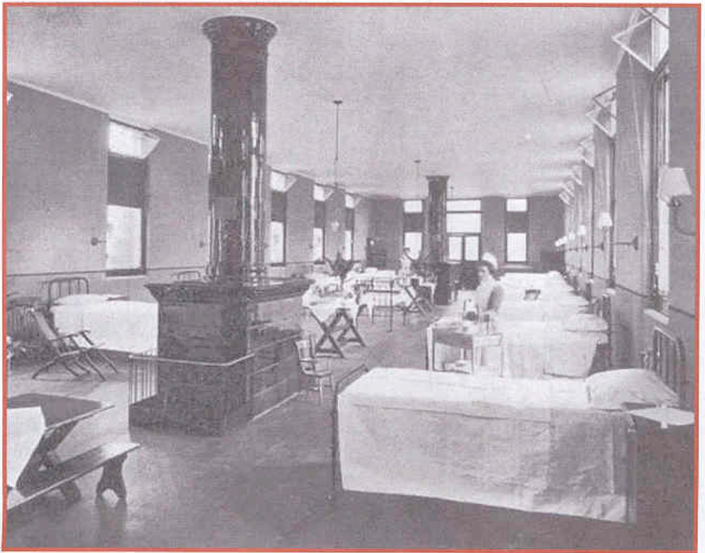
Scarlet Fever Ward [CAC, fig.113] Hospital built 1906, notice the two sets of heating apparatus.
