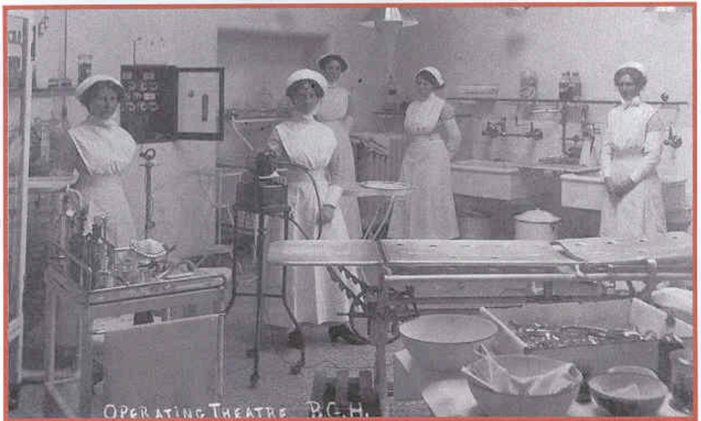
Operating Theatre, Bristol General Hospital, 1907 [MPH, 99] Radiator in far corner; lighting switches in wall cabinet behind assistant on left.
