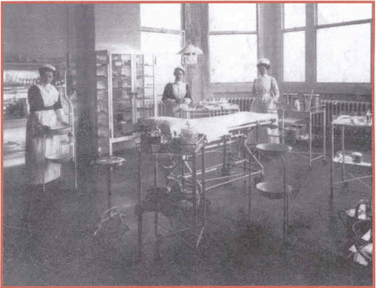
Operating Theatre in King Edward VII Hospital at Windsor, 1909 [CAC, fig.30] Opened in 1909 with 50 beds, architect for the steel-framed building A W West, cost £25000. Heating by under-window radiators with opening windows.
