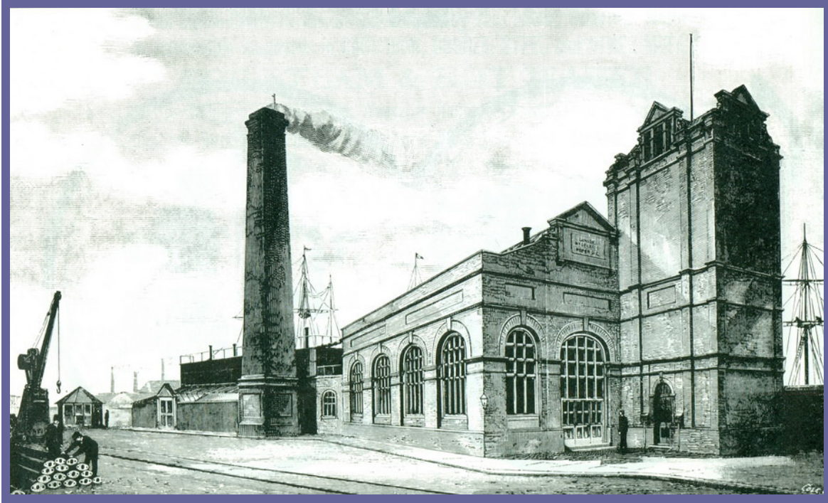
The London Hydraulic Power Company's Station, Wapping, 1893
