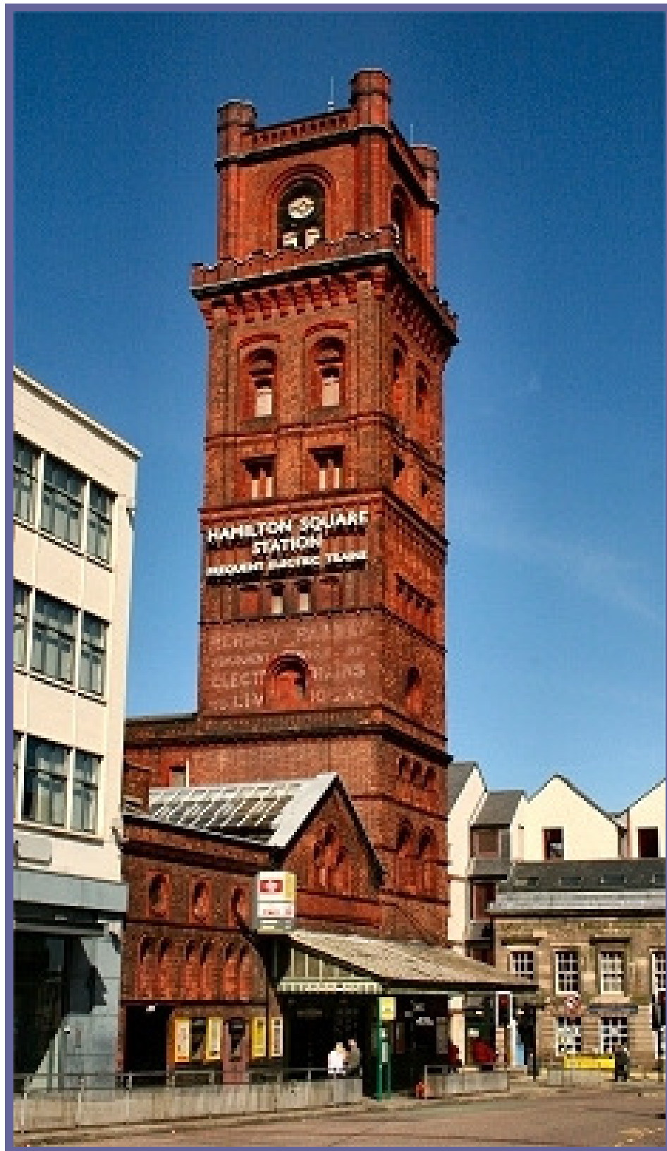
Hydraulic Tower which once powered the lifts at Liverpool's Hamilton Square Railway Station ( allertonoak.com )
