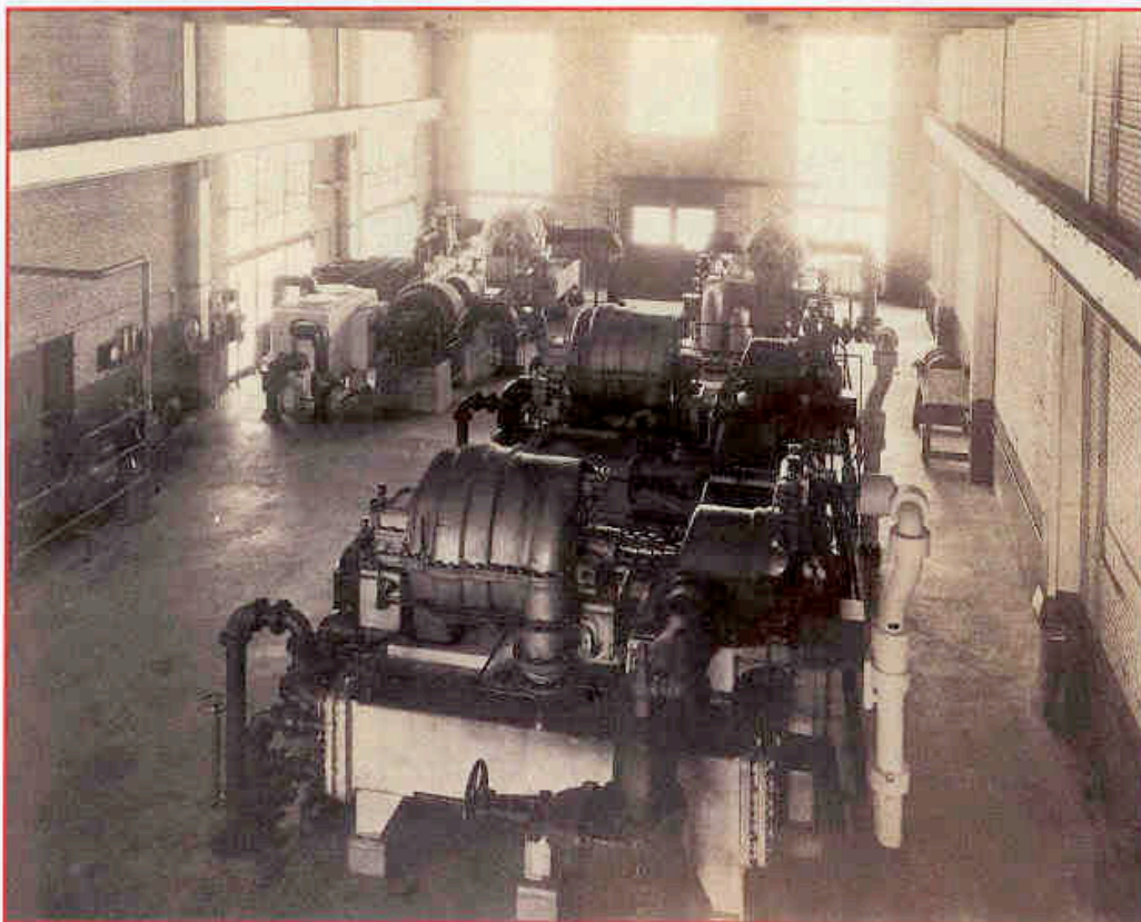
Carrier centrifugal chillers, Wm F Schraft & Sons, Boston, 1923 [Heritage Group Collection, 00586]
