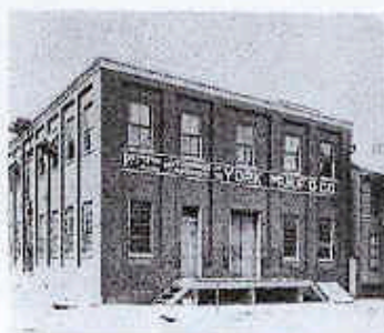
FIRST HOME OF YORK ON PENN STREET, YORK, PA. THIS SMALL BUILDING LATER BECAME THE PATTERN SHOP.
