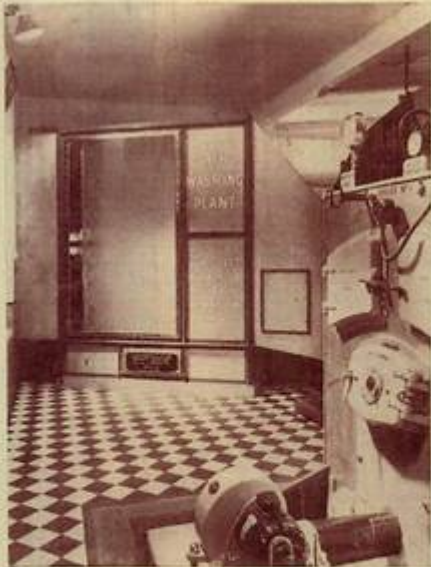
Air Washing Plant.
