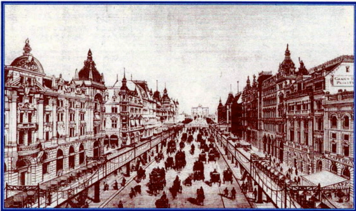
Proposal for a Stepped Platform Railway for (possibly) New York [ Scientific American , 26, iv, 1890]
