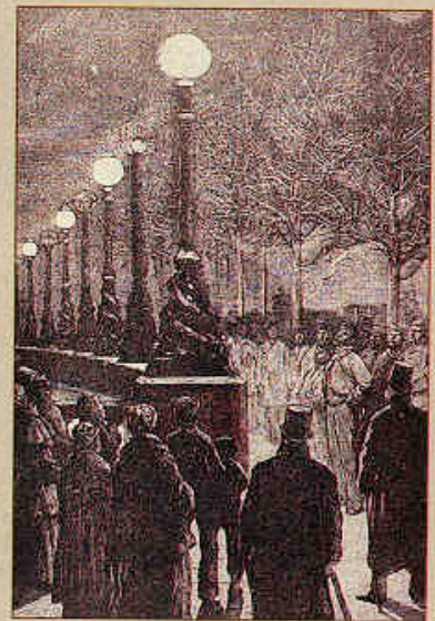
Fig 18: Jablochhoff candles used to illuminate the Victoria Embankment (1878). Wood engraving from The Graphic (4 January 1879).
