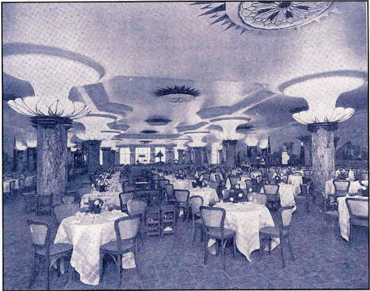
J Lyons Restaurant, Oxford Street Corner House, London. Air conditioned by CEC [HVE, August 1928, 48]
