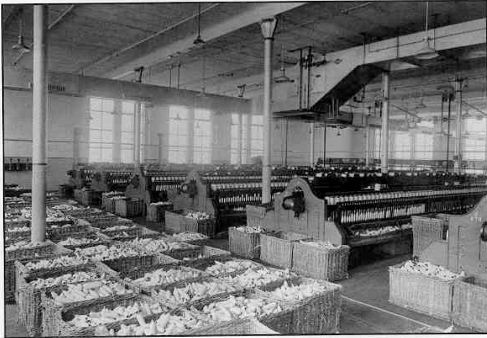
Air conditioning Sewing Cotton Co Ltd, Stanhill Ring Mill, c.1950 [P7-14].
