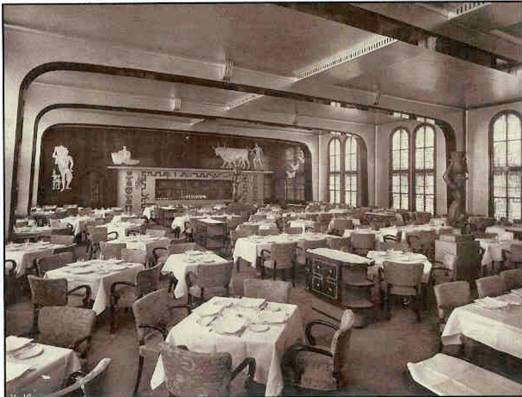
Air conditioned Dining Saloon on "SS Victoria," 1930 [P-657].
