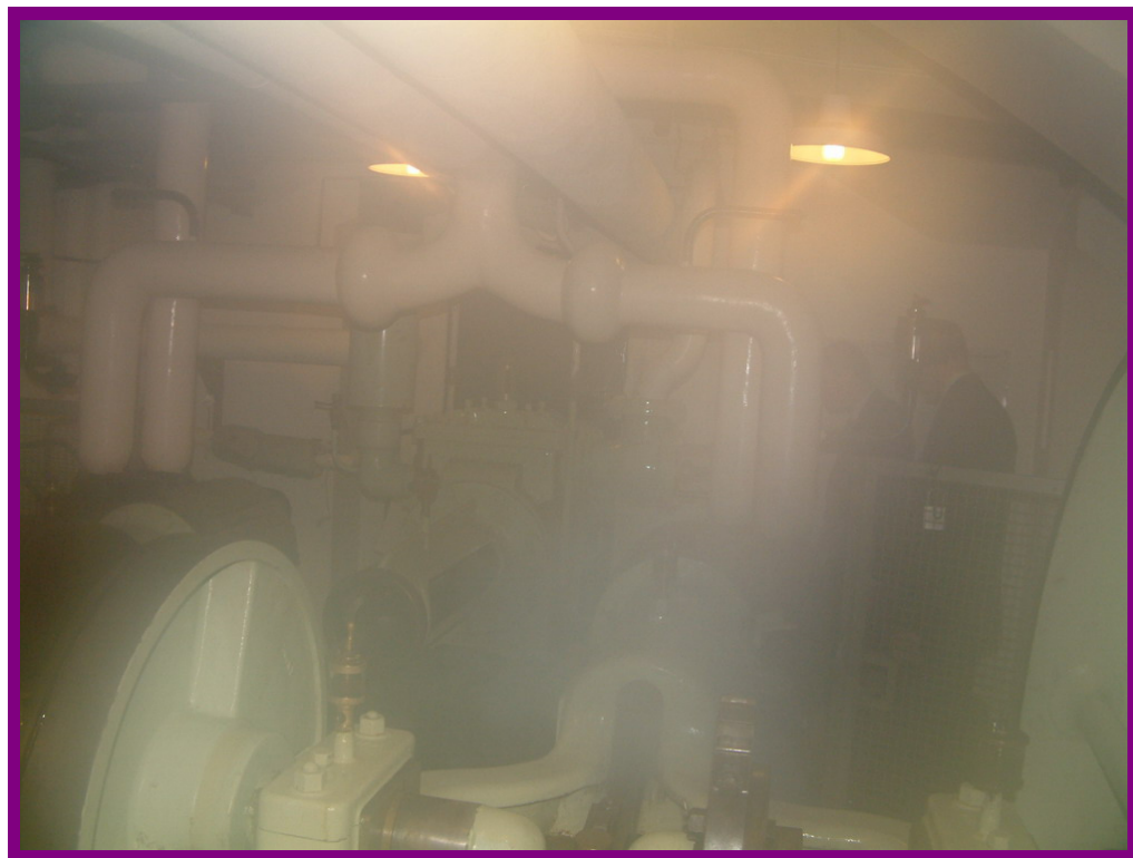
At the Palace of Westminster: the original Marshall Steam-Engine Compressor once used to operate the Shone Ejectors, still in working order.
