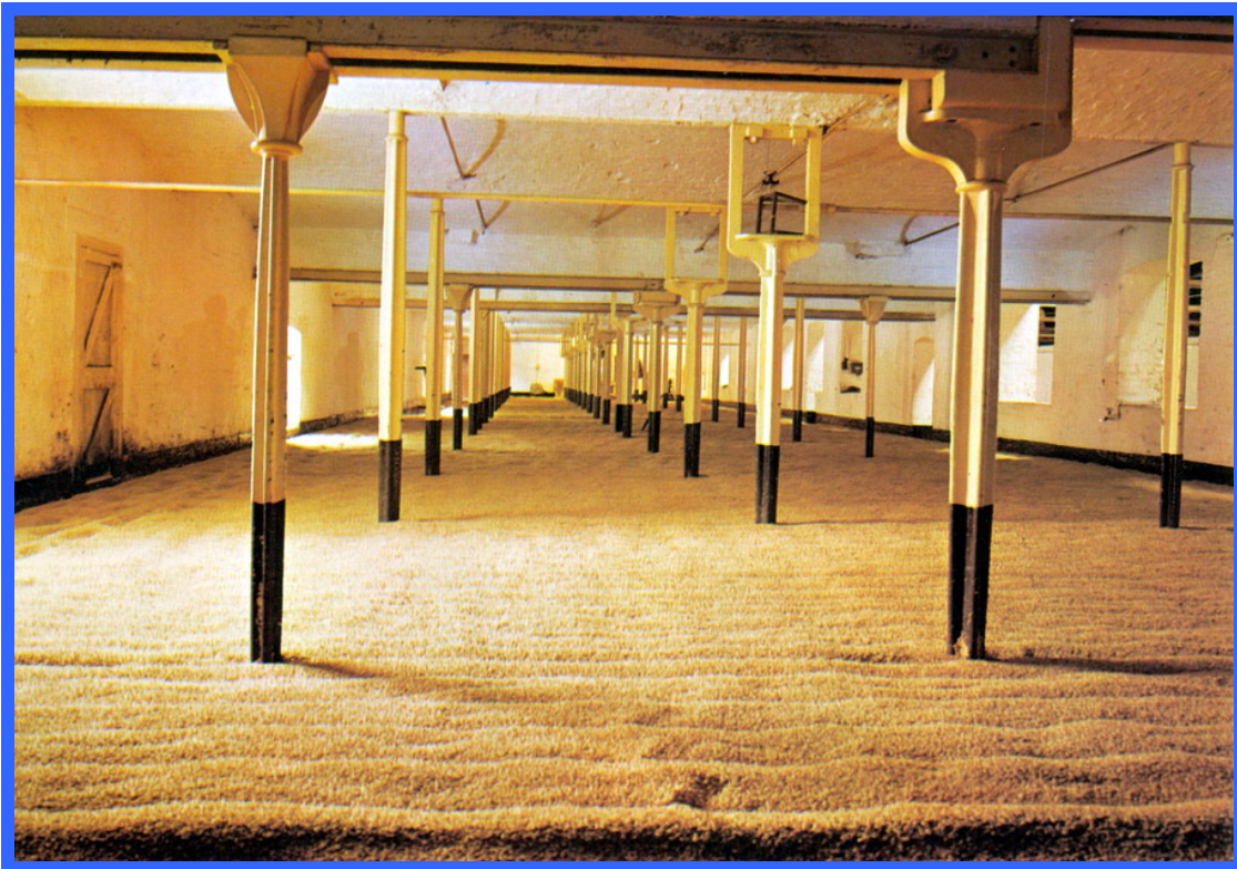
The first iron-framed factory in the world built for the flax-spinning mill of Benyon, Benyon & Bage, Ditherington, Shrewsbury, 1796 “The Archaeology of the Industrial Revolution,” Brian Bracegirdle, 1974 (CIBSE Heritage Group Collection)
