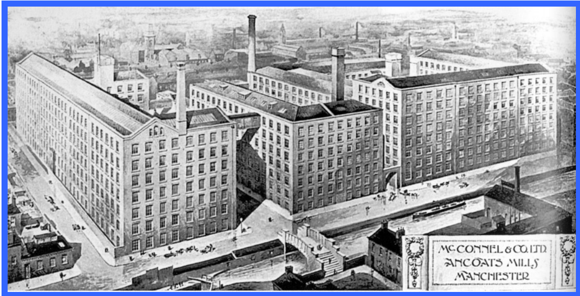
McConnel & Kennedy's early mills, built 1798-1826 by the Rochdale Canal in Ancoats (Williams & Farne)
