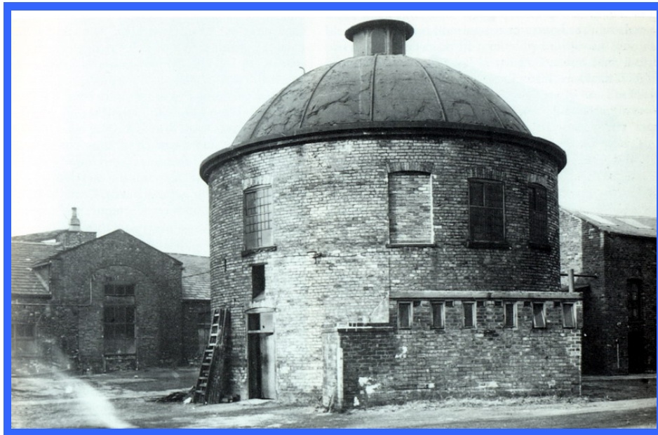
Gas Plant and Gas Holder House at Bean Ing Mills, originally by Boulton & Watt c.1810 but superseded in 1831 (Giles & Goodall)
