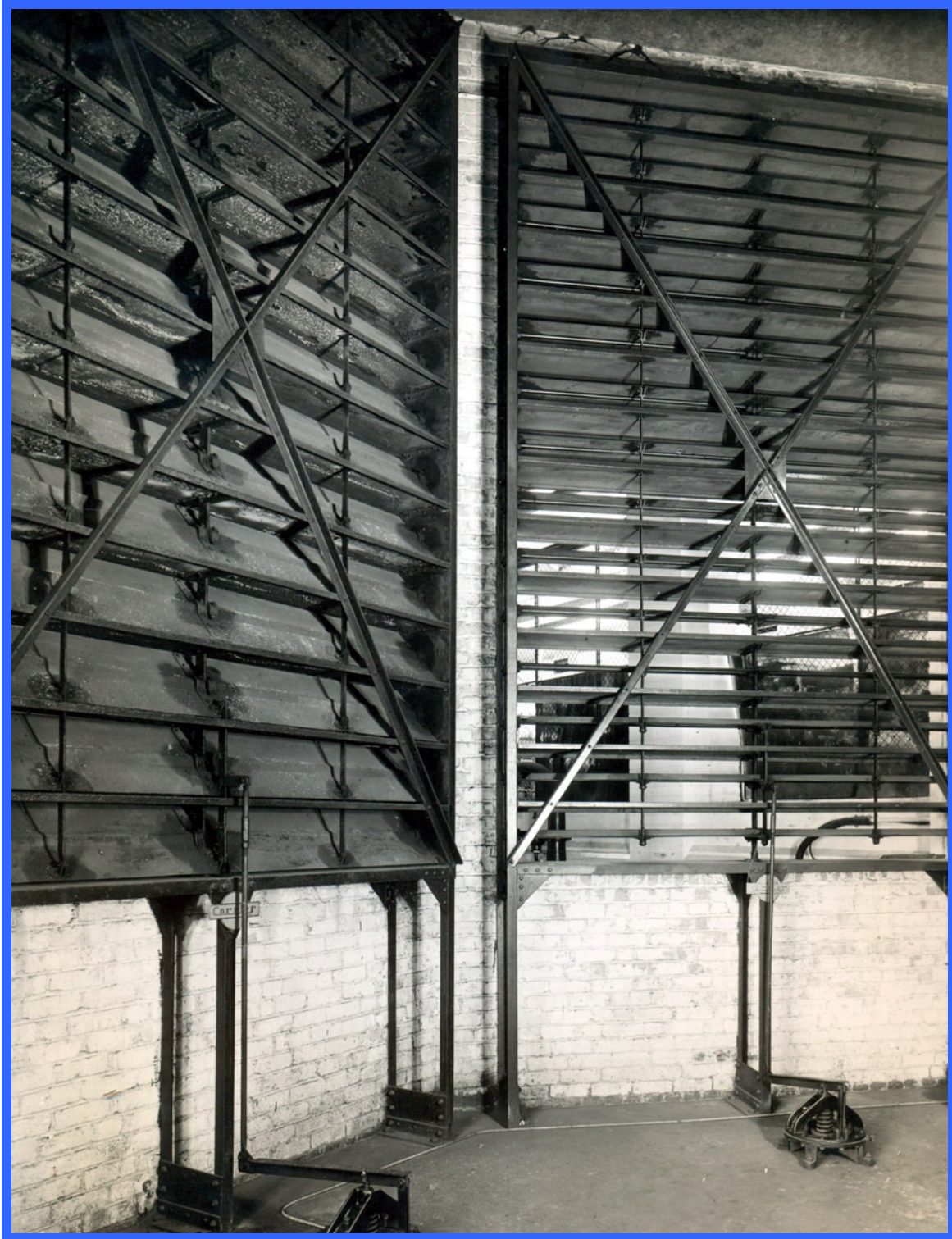
Carrier system of mixing dampers for Weaving Shed at Bedford Mill for Courtaulds of Leigh, July 1949 (CIBSE Heritage Group Collection)
