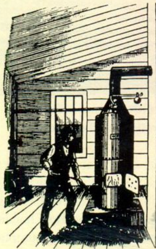
FIG. 170. THE BOILER BEFORE EXPLOSION.
