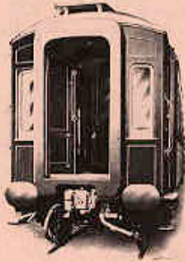
Combination Automatic Door and Vestibule.
