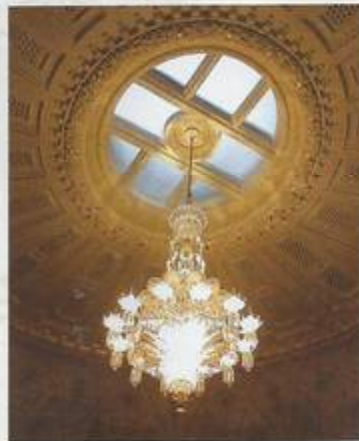
Figure 2: Concert Room ceiling showing roof-light and air outlets
