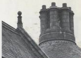
Phipson's combined extract stack and fireplace chimneys at the Liverpool Royal Infirmary
