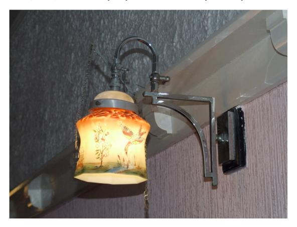
The adaptation of older, often originally upright open flame fixtures, is another common alteration used to make the earlier fixture more suited to the level of illumination achieved by the later fixtures. Maurice has a lovely pair of Victorian swivel arm wall brackets onto which he grafted an inverted No.3 burner with pilot and lever cock using a bend we made for him at Sugg Lighting. These two flank the dining room fireplace in which as you can see there is a splendid ancient gas fire.
