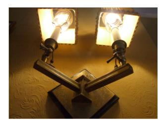
Although the house was built in the era of gas light, the fixtures have all been installed by Maurice assisted by his installer in more recent times. There are many 30's style chrome plated fixtures of which this 'spaceship' style, below, is a classic with permanent pilot and switched remotely from beside the bed! Somewhat unromantically, they are in fact simply G89837, part of the Pool-Light Series made by Veritas.
