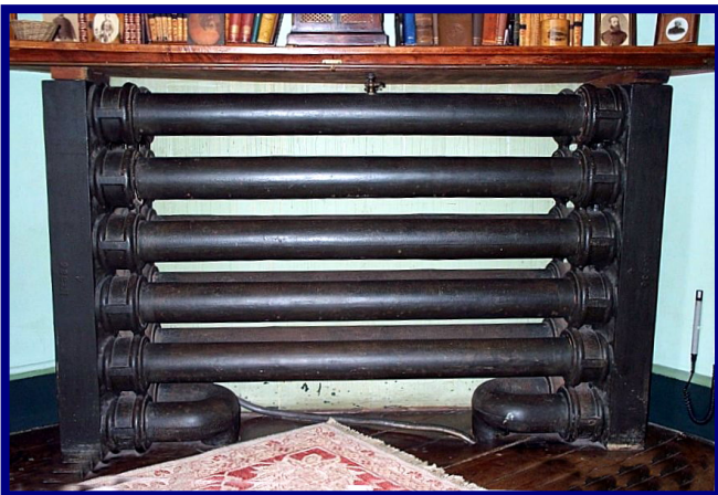
LPHW cast iron pipe coil heater
