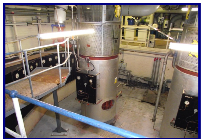
Sulzer 6.6 kV off-peak electrode boilers serving the LPHW thermal storage heating system
