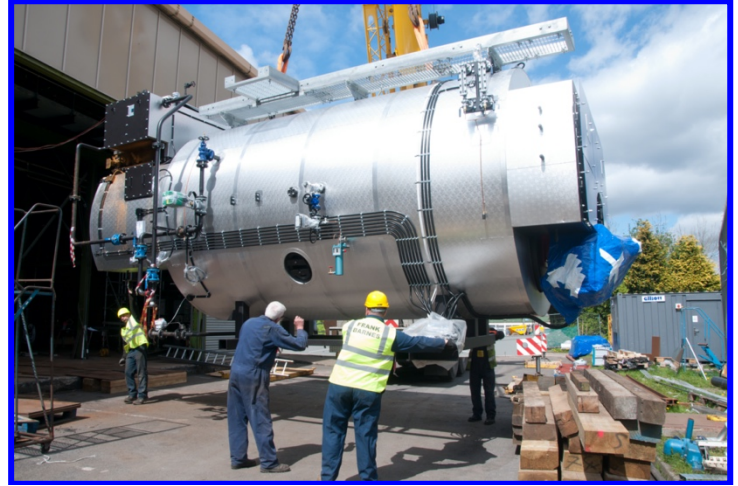
Installing modern boiler for Bolton NHS 2017
