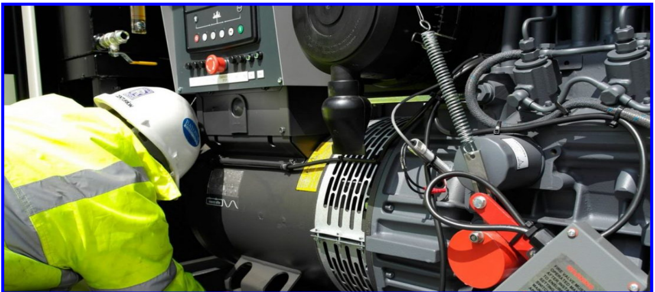
Standby Diesel Electric Generator Set
