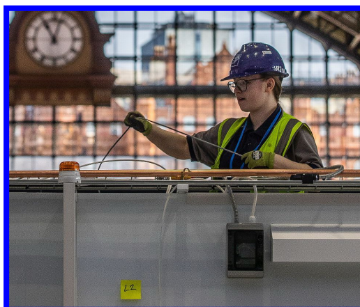
Completing electric wiring
