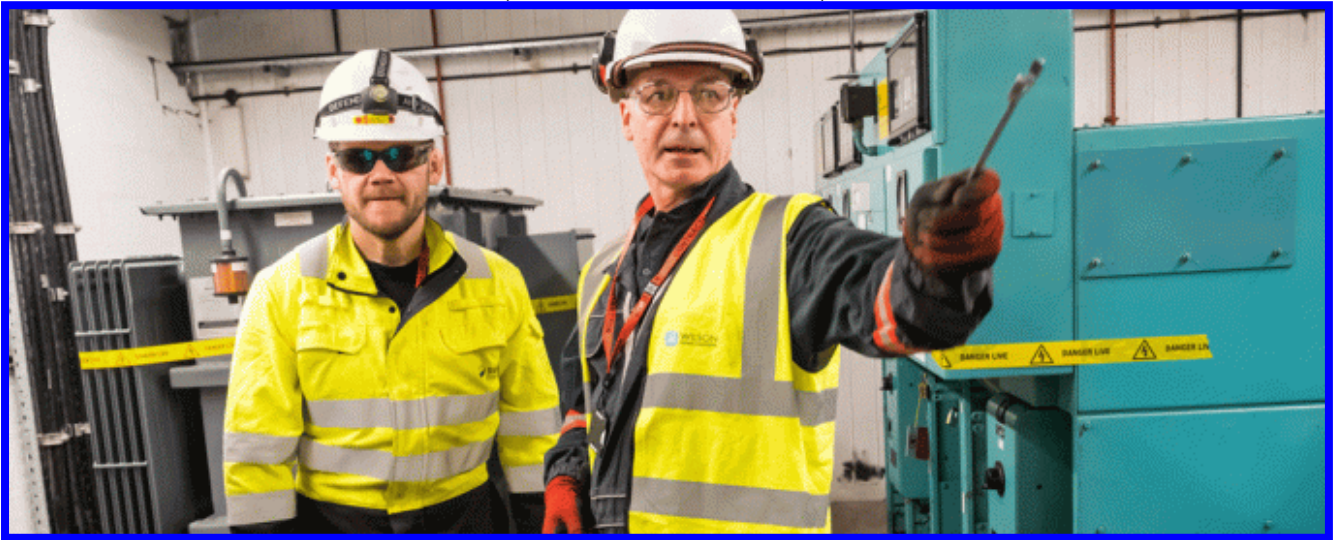
Energy consumption monitoring and control
