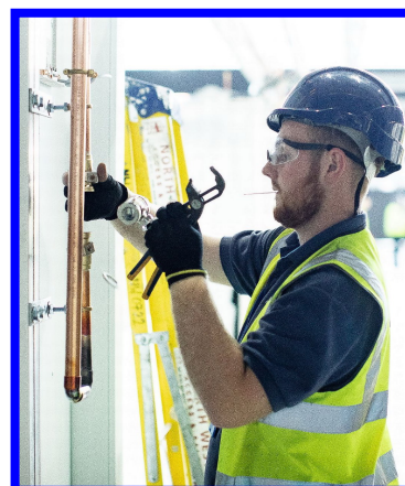
Fitting oxygen pipes
