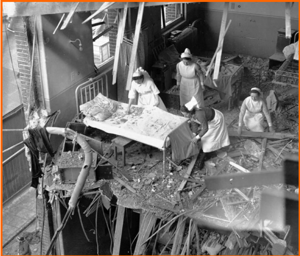
Inspecting damage at St Peter's Hospital Stepney, East London 19 April 1941
