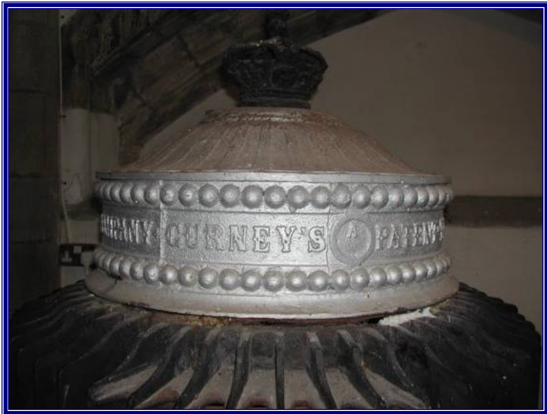
Gurney stove in St Nicholas Church, Grosmont, Monmouthshire
