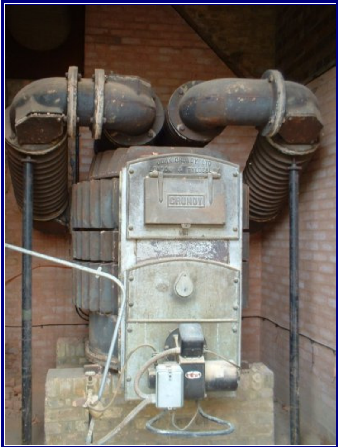
Oil-fired Grundy heater St Barnabas Church, Epsom (now destroyed)
