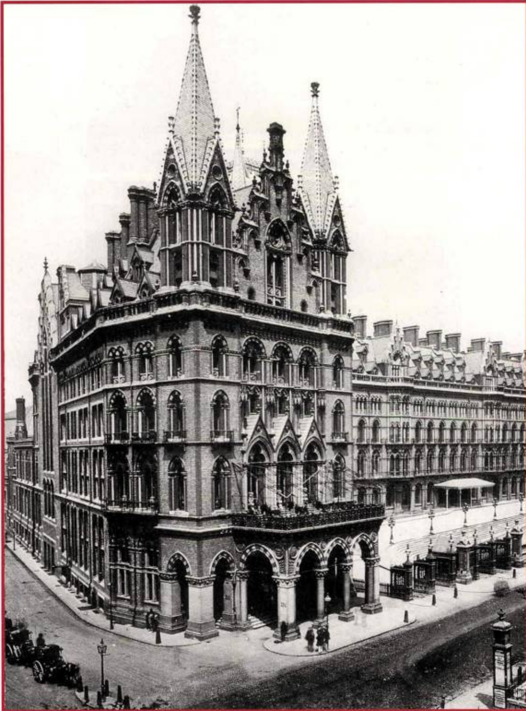
1874 Midland Grand Hotel (St Pancras) London Heating for the Hotel and Station by G N Haden & Sons Contract values £4072 16s 0d and £968 12s 0d The architect was Sir George Gilbert Scott
