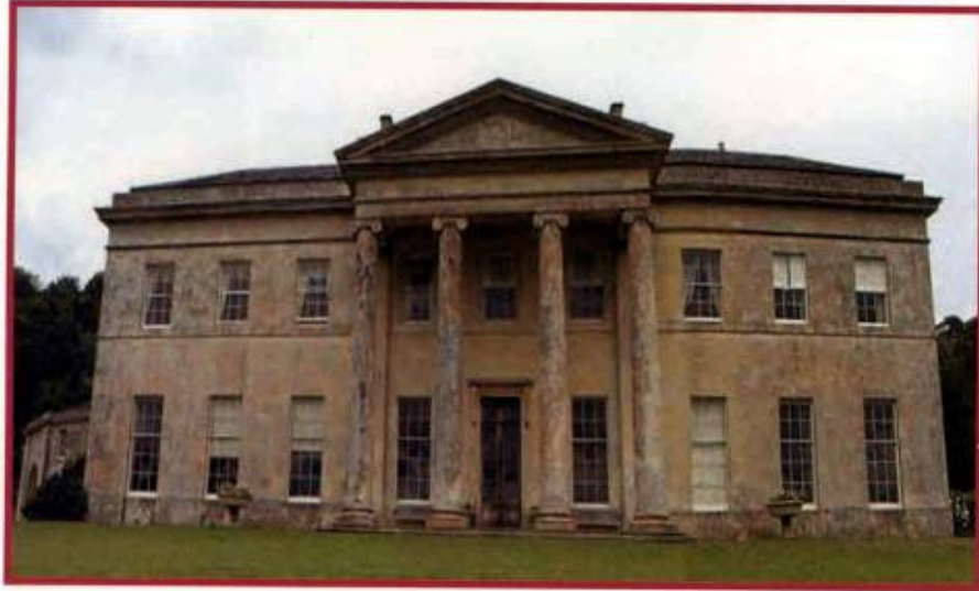
Dinton House (now Philipps House) Dinton Park, Wiltshire Architect Jeffry Wyattville [FJF]
