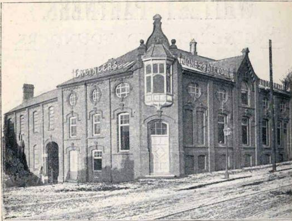
MESSRS. JONES & ATTWOOD'S ENGINEERING WORKS (OFFICE BLOCK).
