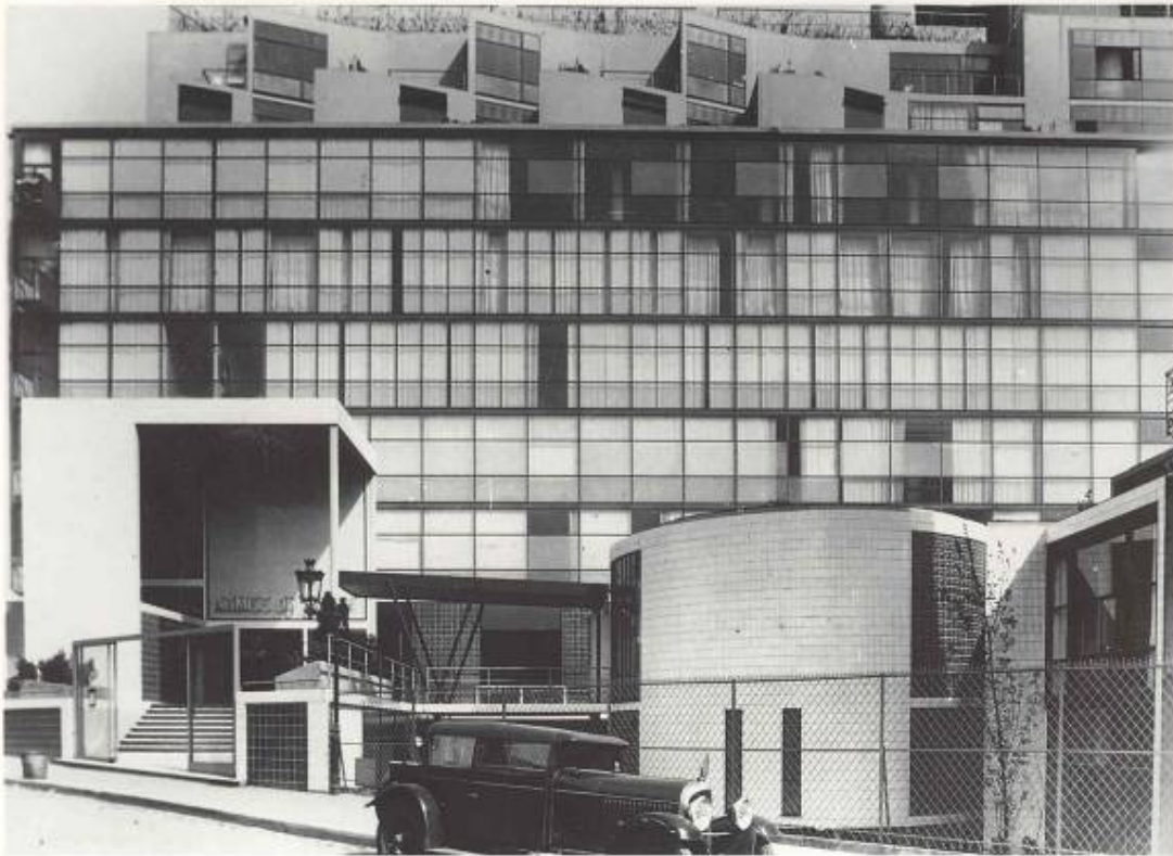
Le Corbusier and Pierre Jeanneret Salvation Army Shelter in Paris, 1929–1933 South front Fondation Le Corbusier, Paris Individual stereometric bodies are placed before the long main building. A bridge leads from the open entrance cube to a cylindrical reception building, a sort of outside concierge's booth with a lounge behind. Dormitories and common rooms initially for 900 and later for up to 1500 homeless lie behind the hermetically-sealed glass façade. A ventilation system was installed which proved wholly unsatisfactory, leaving the rooms to reach hot-house temperatures in summer.
