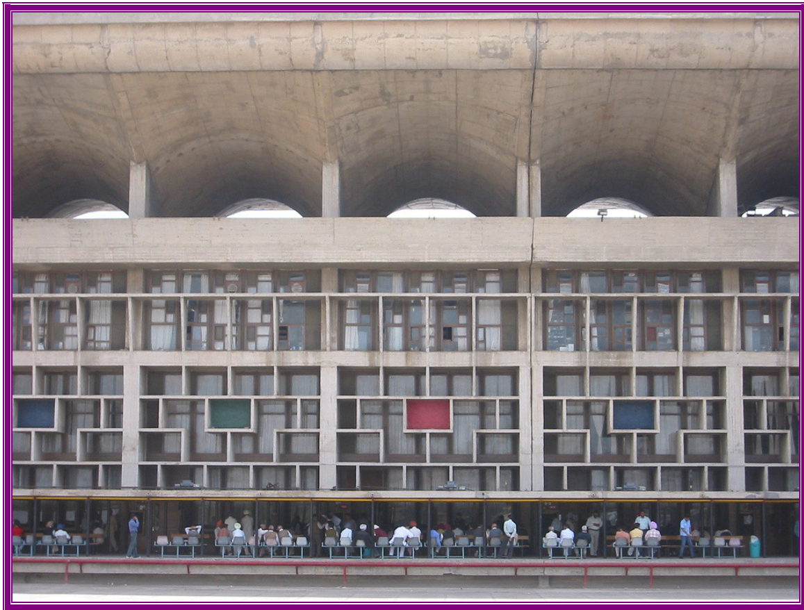
The High Court, Chandigarh, India, 1956, provided with Solar Screens and Natural Ventilation
