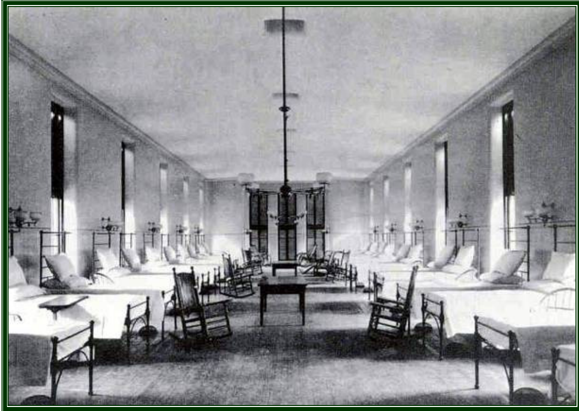
John Hopkins Hospital This Common Ward is fitted with "blacksmith beds" featuring ventilating ducts under each bed
