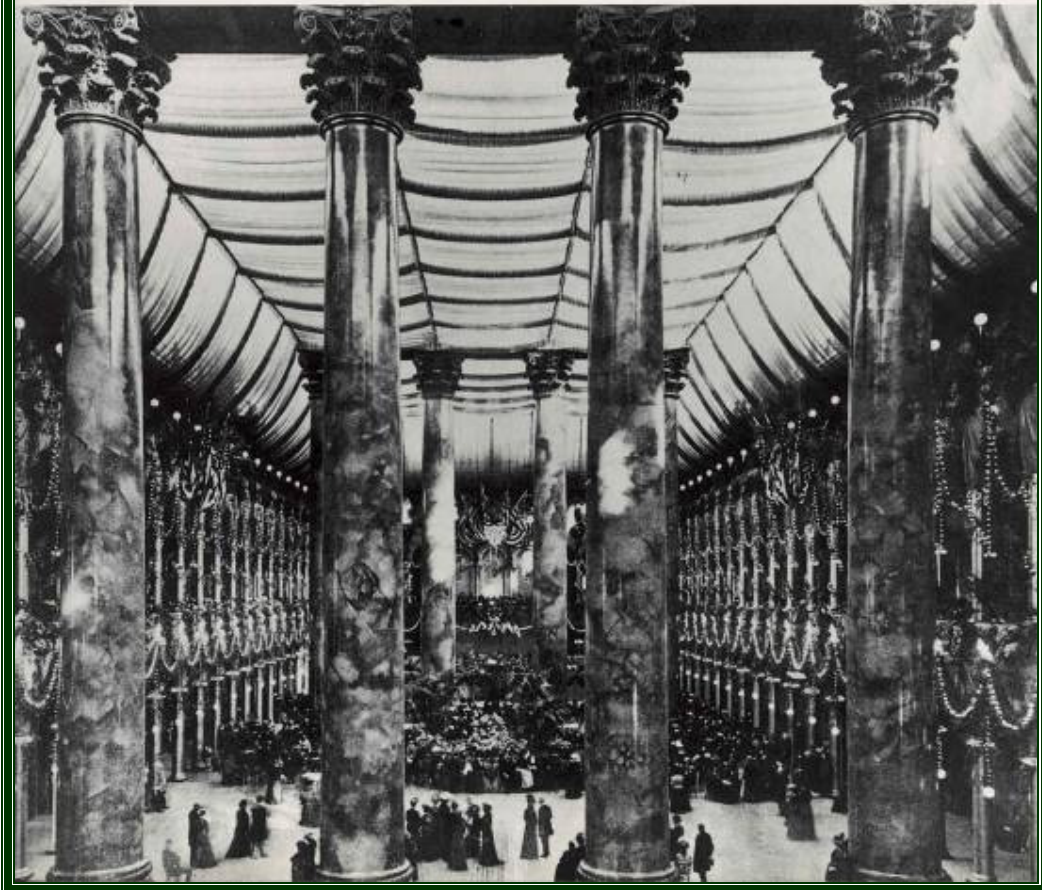
The Old Pensions Building ("Works in Progress," Alvin Rosenbaum, 1994)
